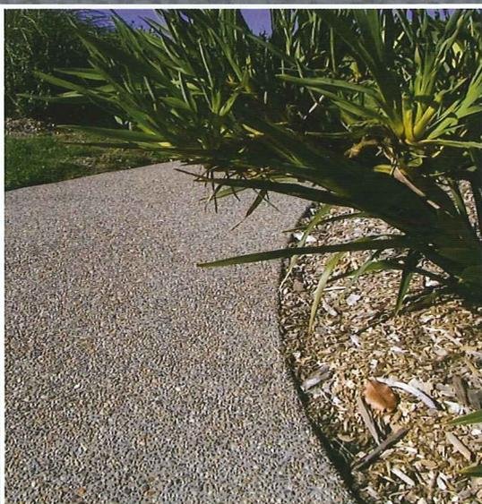
**COLOUR:** Colour is an architectural tool and can bring a project to life. The desired colour of the finished concrete can be achieved in a number of ways. The most common method is to colour the cement paste (cement and water) using a mineral oxide pigment. Alternatively, a decorative aggregate can be selected for a particular effect.
