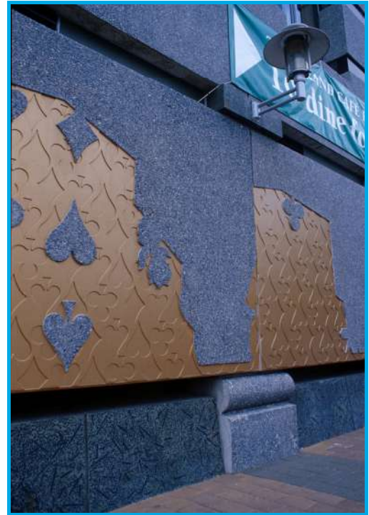
Christchurch Casino, Christchurch. Precast concrete. Exposed aggregate and polished concrete.
