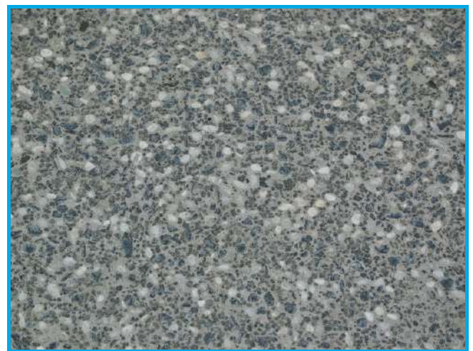
Residential Driveway. Cast in-situ with exposed aggregate.
