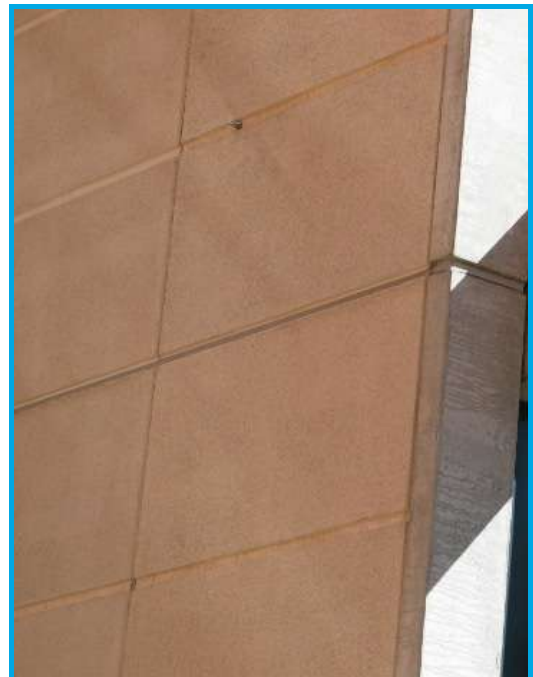
Wellington Public Library, Wellington. Precast concrete with exposed aggregate.
