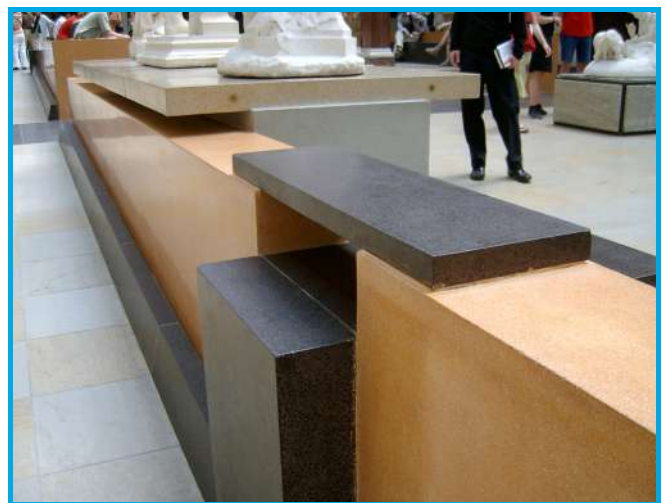
Musee D'Orsay, France. Precast concrete – coloured and polished.
