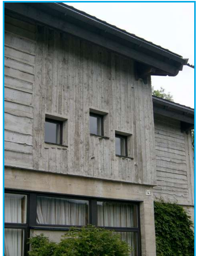
Mølster Museum, Voss, Norway. Board formed cast in-situ concrete.
