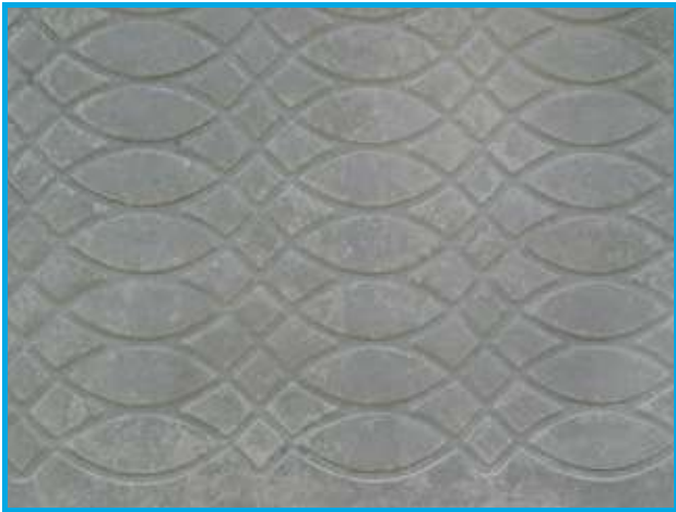
St. Joseph’s Church, Wellington. Precast concrete using form liners.
