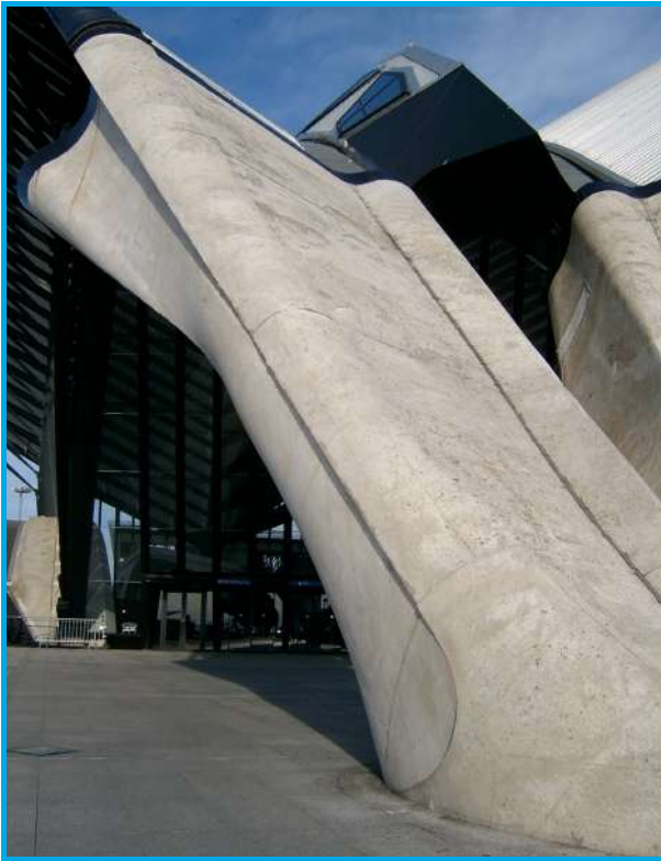
Lyons TGV Station, France. Cast in-situ concrete.
