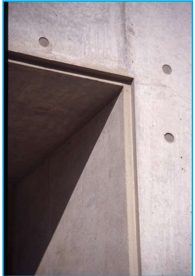
St Paul's Apartments, Wellington. Precast concrete using form liner.
