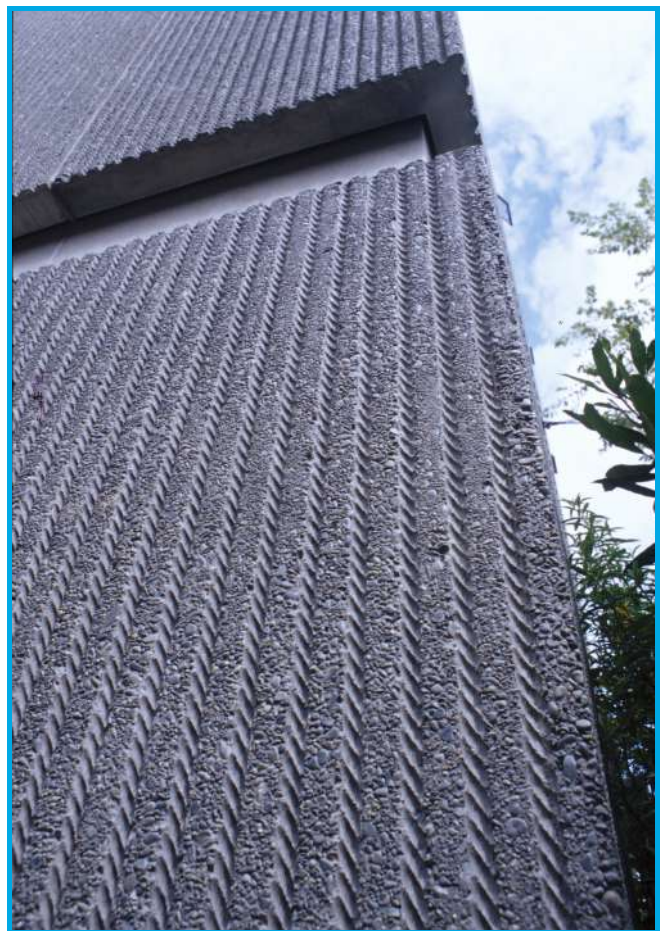
Christchurch Public Hospital, Christchurch.
