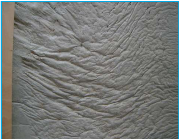
Plastic Ruffled Appearance – Lyon University. Cast in-situ concrete using form liners.
